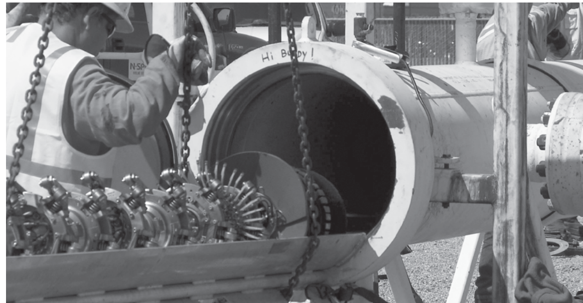
The in-line inspection tool, known as a smart pig, will provide finely detailed data on the condition of a gas transmission pipeline.
